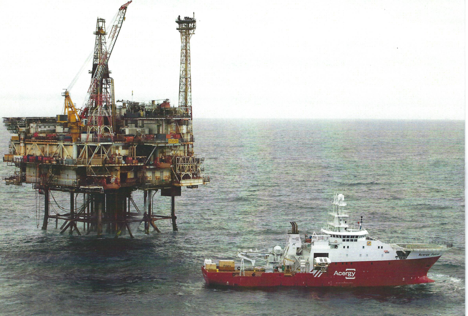
Apache's North Sea Bravo platform. After Apache purchased BP's 96% share in the Forties field in 2003, it reanalyzed and re-evaluated old geophysical data and found a further 800 million bbl. Mining this data was possible with SEG's open data storage standards allowing upward compatibility from old media to a new medium. Photo courtesy of Apache Corporation.
