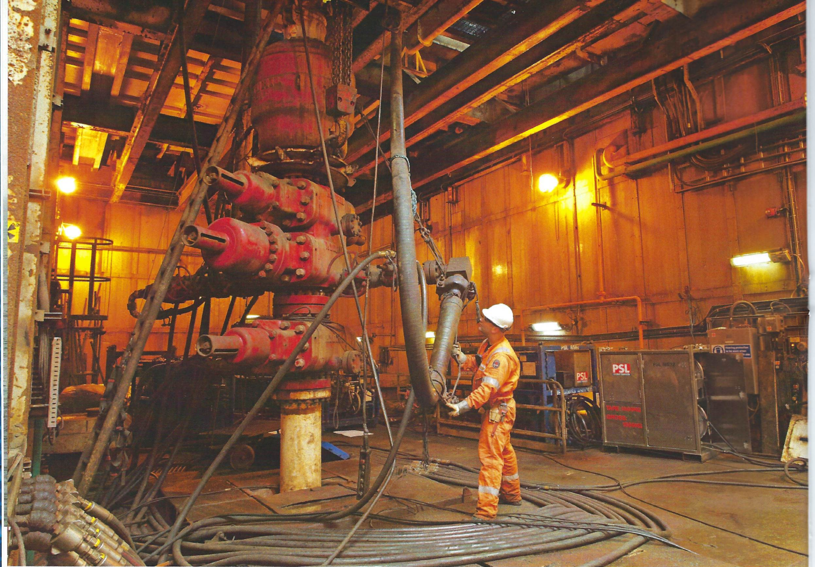
Apache's North Sea Charlie platform, located in the Forties field, along with its Alpha, Bravo, Delta, and Echo platforms. Rejuvenation of the Forties field relied on plumbing old geophysical data, which was possible with SEG's open data storage standards allowing upward compatibility from old media to a new medium. Photo courtesy of Apache Corporation.
